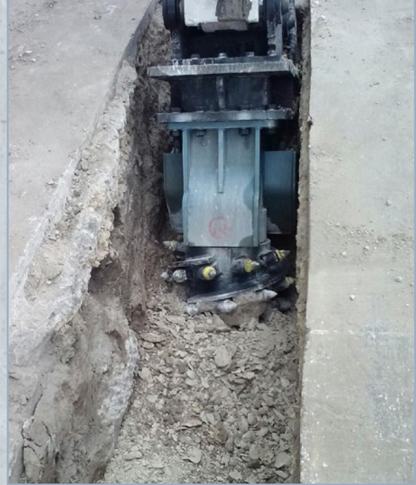
TC20 in a utility project
